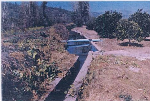
▲ Secondary canal and division works
