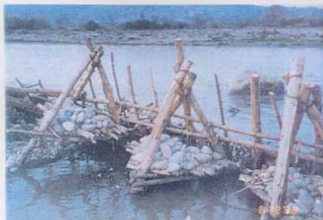
▲ Traditional intake facilities (Downstream of the Mapocho River)
