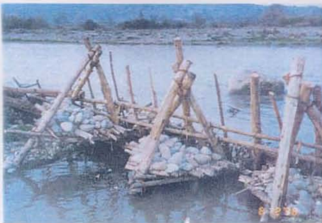
▲ Traditional intake facilities (Downstream of the Mapocho River)
