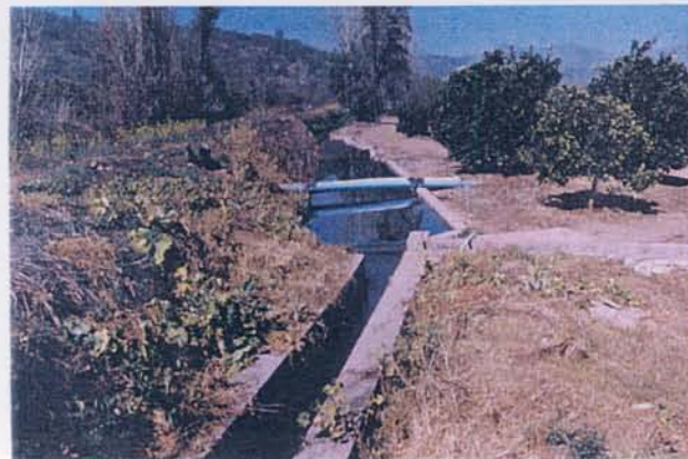
▲ Secondary canal and division works
