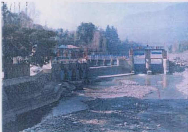
▲ Intake facilities of the first section of the Maipo River (Obra head works) Left; San Carlos canal for agricultural use, Right; intake canal for water supply managed by EMOS
