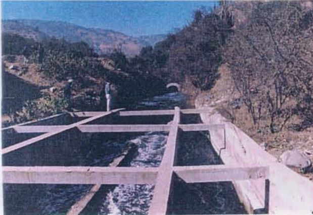
▲ Division works after the exit of the tunnel of Mallarauco canal
