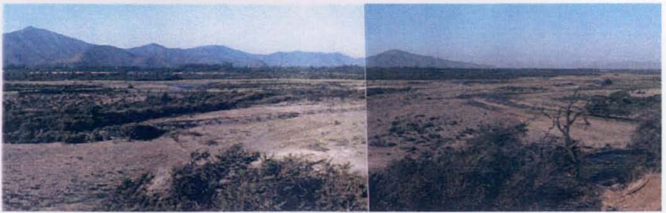
▲Proposed site for integrated intake weir in the upper stream (The third section of the Maipo River)
